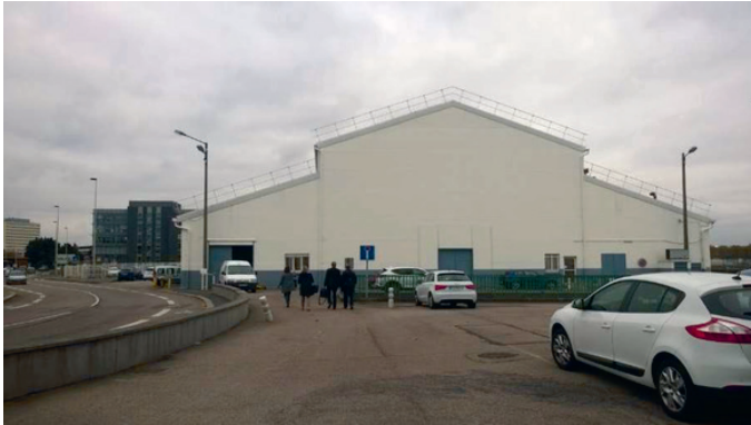
Renovated Hangar at Le Havre
