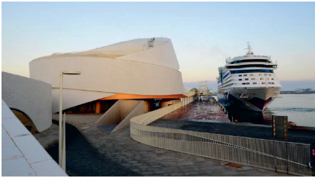
New South Terminal at Porto
