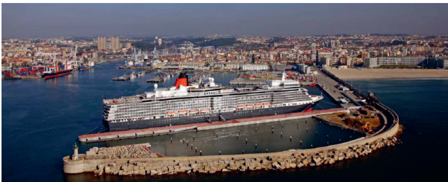
New Berth prior to construction of terminal building 9
